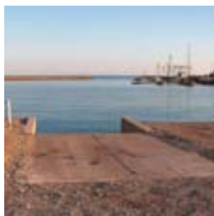
4 Roomassaare sadam. Betoonkate. N 58°13'04,6" E 022°30'19,5"
