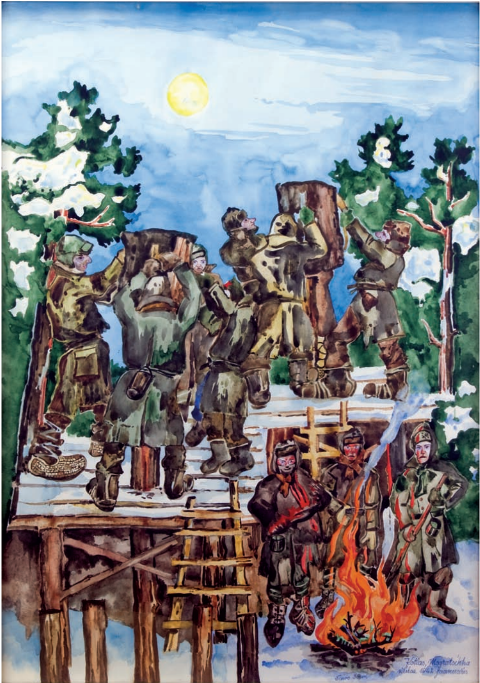
Vantidega palkide rammimine külmunud maasse. Mogsratsihka küla, jaanuar 1942. Ramming beams with supports into frozen ground. Mogsratsihka village, January 1942.
