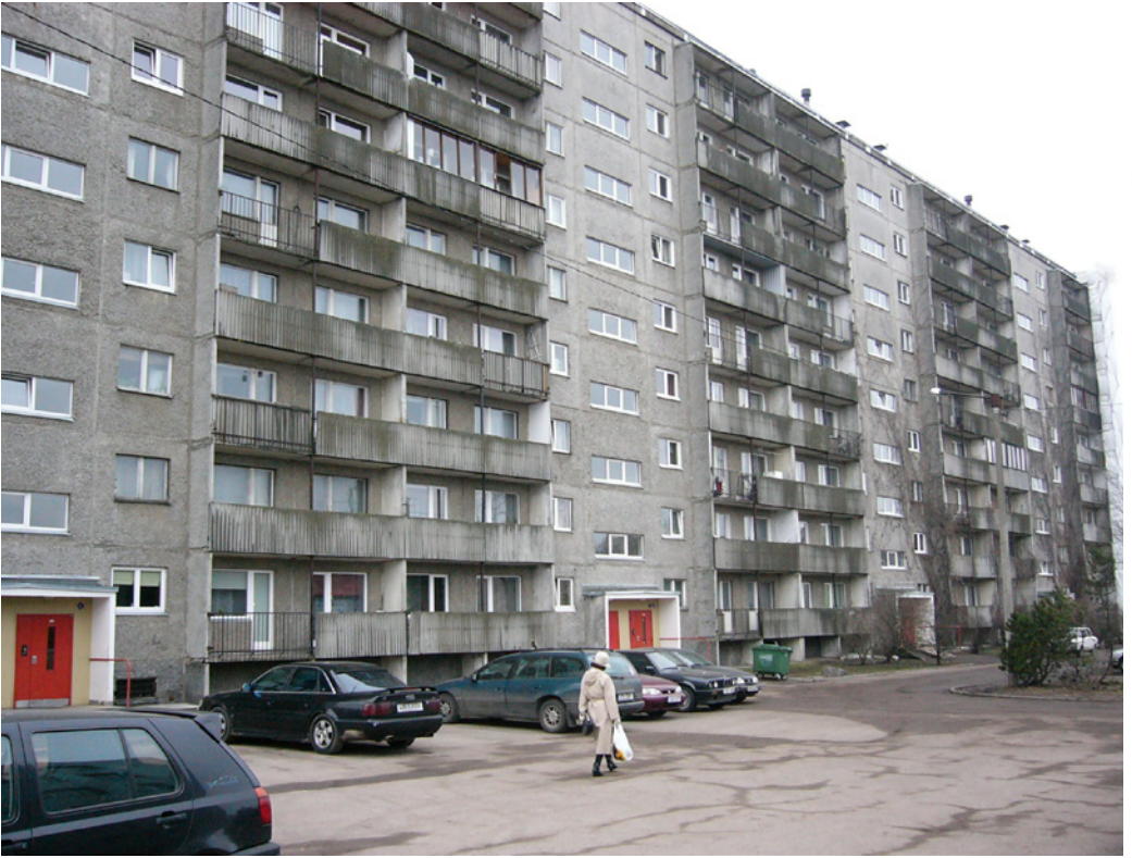
Figure 8 Apartment building in Mustamäe, Tallinn, Estonia, 1960s. Photograph by author, 2007.
