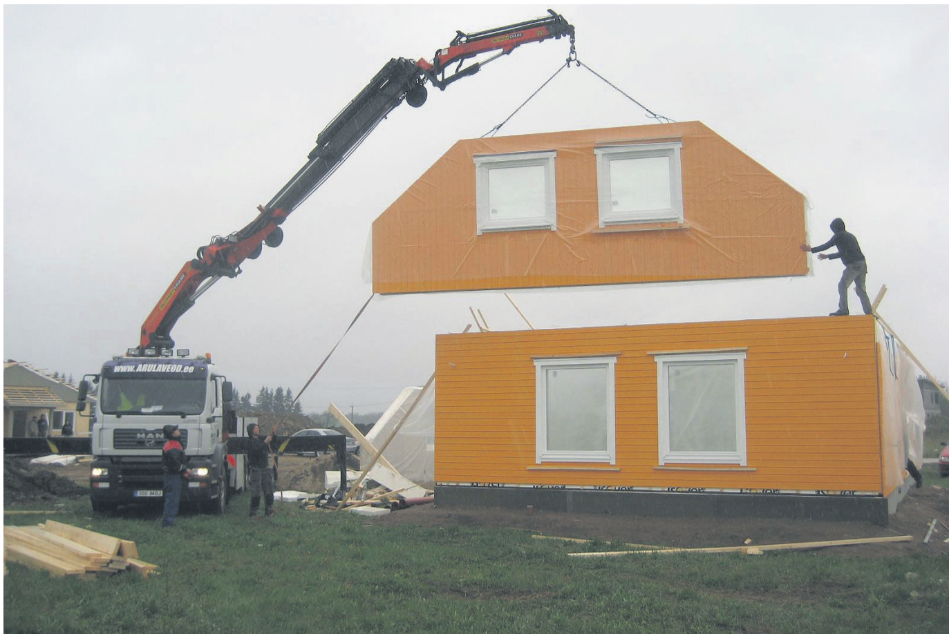
Elementide paigaldamine objektil
