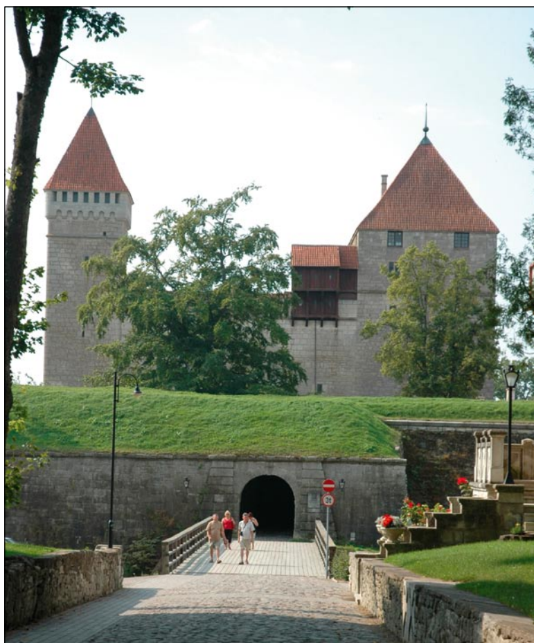
Fig. C26. Front view of the Kuressaare castle. Photo by O. Hints.
