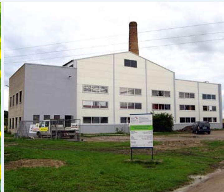
A boiler plant in Lihula working on herbaceous biomass
