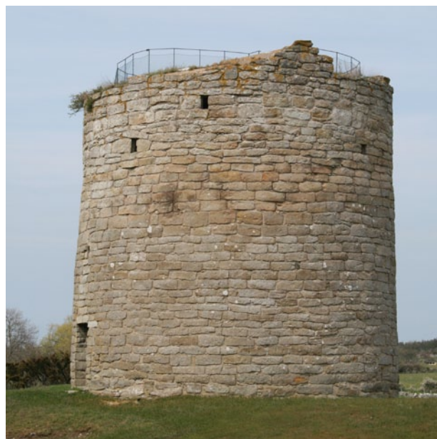
The Sunde medieval church lies in the far south of Gotland. This defence tower is situated near the church, and it gives the place a certain significance. The tower is one of the oldest buildings in Gotland, dating back to around 1000. The Sunde church defence tower, Gotland. Photo: Joakim Hansson.
