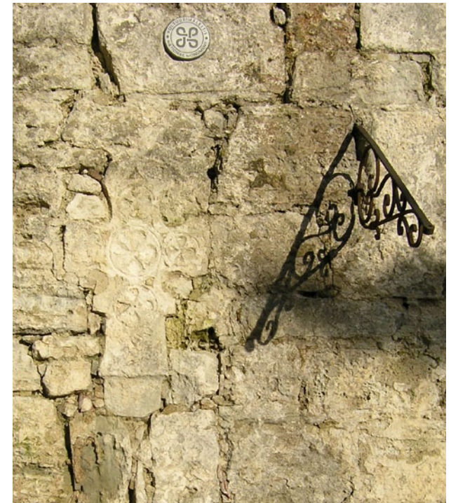
The materials used in building churches have often been reused. A medieval stone cross used as part of the buttress at the Kaarma church, Estonia. Photo: Kaire Tooming.
