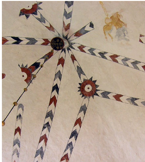
All historical layers are important for the integrity of the building. None should be preferred over others. Three different layers of vault paintings, dating from the late Middle Ages to the Baroque, were found and displayed during conservation work in the Martna church, Estonia. Photo: Kaire Tooming.
