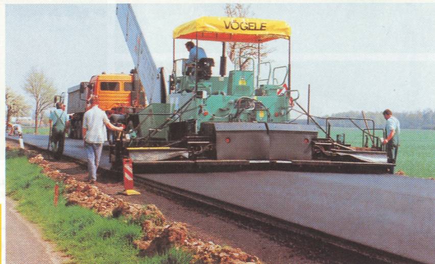
Paving asphalt base 11 cm deep and 6m wide for highroad.
