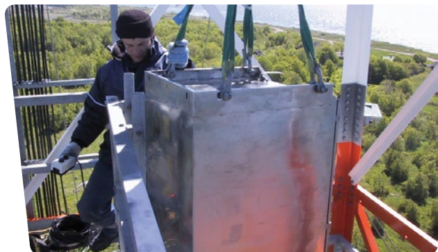
Transceiver's installation to an antenna for GOFREP system
