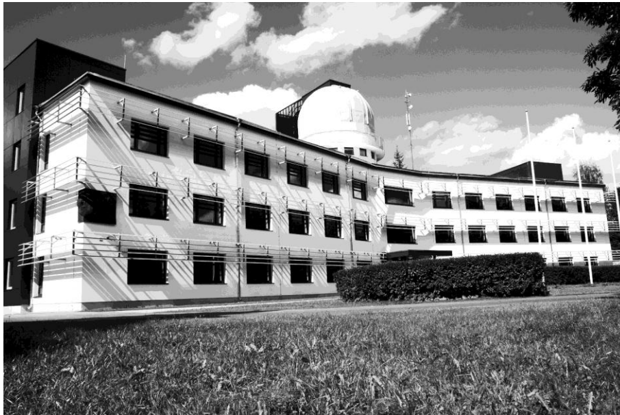
Renovated building of the Observatory, photo by Kalju Annuk
