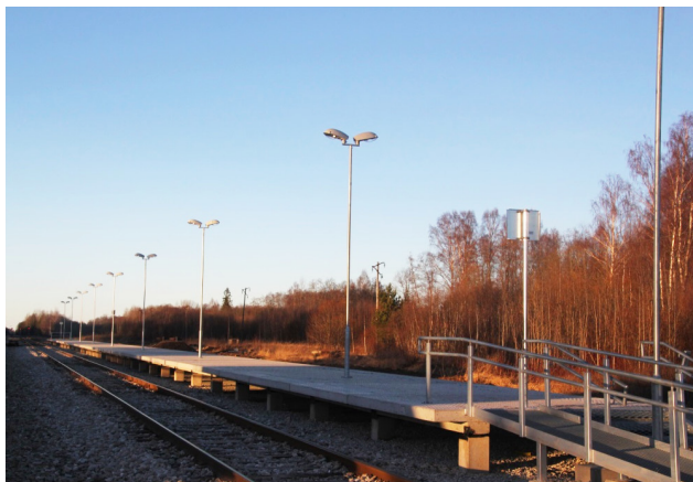
Lelle waiting platform between roads completed in 2013
