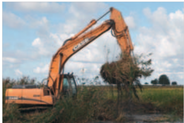
Photo 6.1.8. Removal of reed and its thick rhizome layer with a digger from the northern shore of the large lagoon of Võiste in 2009.
