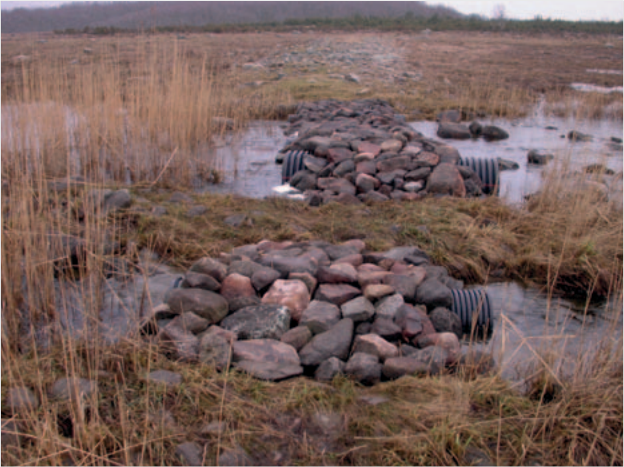
Photo 6.2.3. Installed culverts in the historic cobblestone dike.
