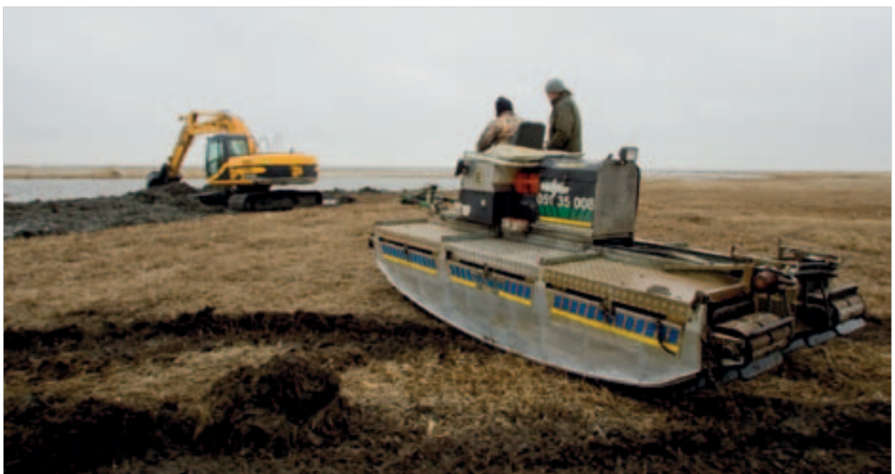
Photo 6.1.6. Spreading of the sediments and plant parts removed from the lagoons to the shores (on the background). On the foreground, a Truxor amphibian tractor.
