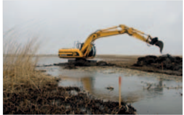
Photo 6.1.5. Restoration of a sea connection channel of a coastal lagoon with a digger
