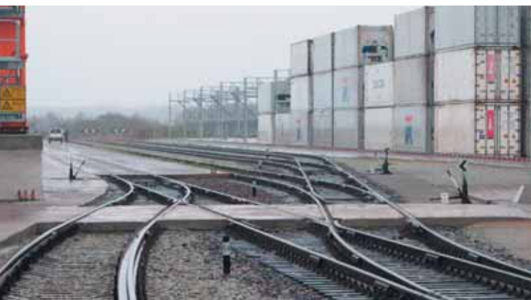
New railways in the Coal Terminal of Muuga
