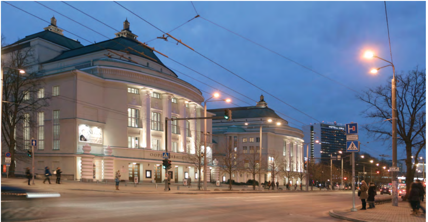
The building of the Estonian National Opera and the Estonia Concert Hall.
