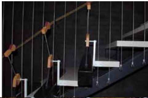
Veronika Valk and Kadri Klementi (architects), Kalle-Priit Pruuden (sculptor), Kalle Tikas (sound designer), Peeter Laurits (artist). Lasva Water Tower Conversion . Estonia, 2006-2009. The main attraction of this building is the piano stairs, which can be played like a musical instrument and lead up to a grass roof viewing platform. This project has helped to restore and strengthen a sense of identity in this remote rural community.
