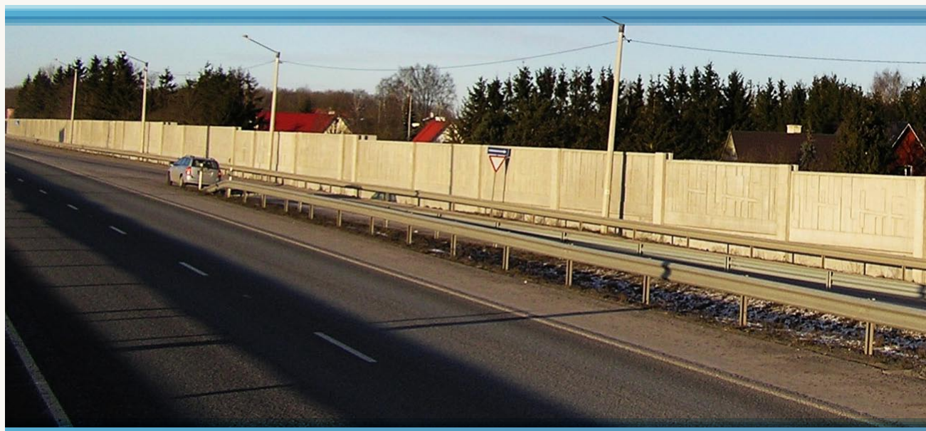
The Pildiküla noise barrier wall, completed in 2007.
