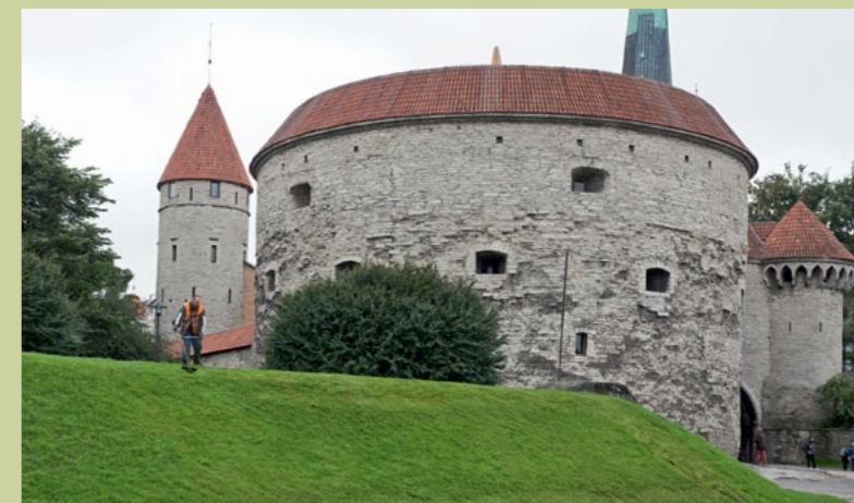
Hooldustööd Paksu Margareeta juures. Maintenance work near Fat Margaret Tower.
